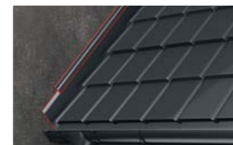
Wall flashing with an expansion strip
