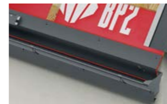
Starting drip-edge flashing for the gutter
